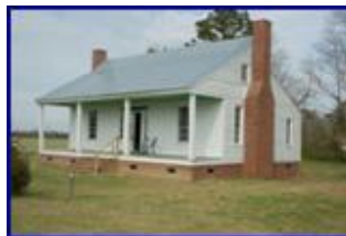
William Phillips House Currently undergoing restoration
