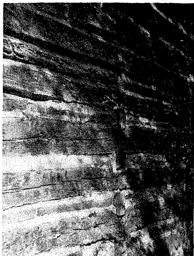
Interior log partition extends to exterior
