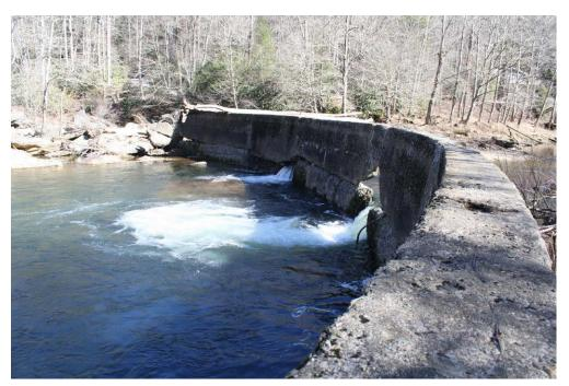
Plate 13.2: Close-up of Shull's Mill Dam (WT0955), showing hole punched in the concrete.
