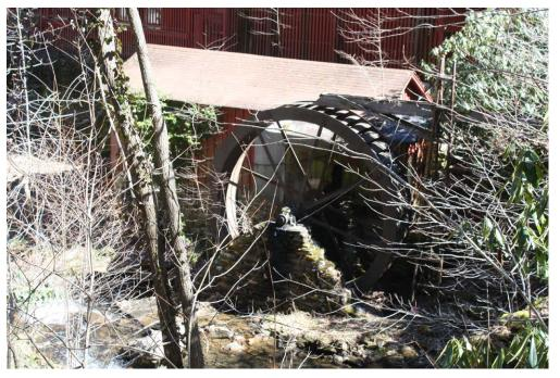
Plate 2.5: Ray Estes Complex (WT0954), small overshot water wheel.
