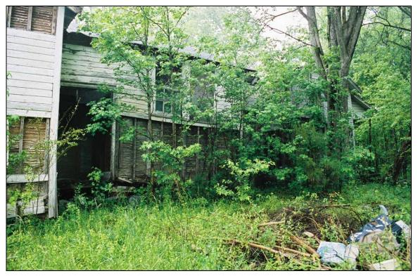
Plate 68. Chestnut School: south front elevation, note loss of weatherboards
