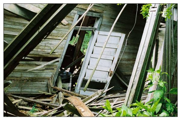
Plate 47. Wimberly School: transom and six-cross-panel door amidst collapsed structure
