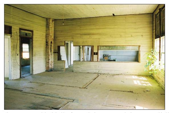
Plate 191. Morgan School: looking from south classroom to north classroom; note blackboard at right center partially lifted up into partition wall
