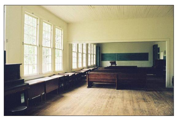
Plate 64. Allen Grove School: interior of the two classrooms; note wood floor, plaster walls, tongue-and-groove ceiling, 9/9 sash, and opening in place of original movable partition wall
