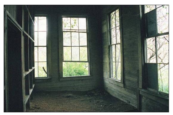
Plate 230. Bunn School: eastern half of industrial room with later-added partition wall at left; windows at right are likely later insertions
