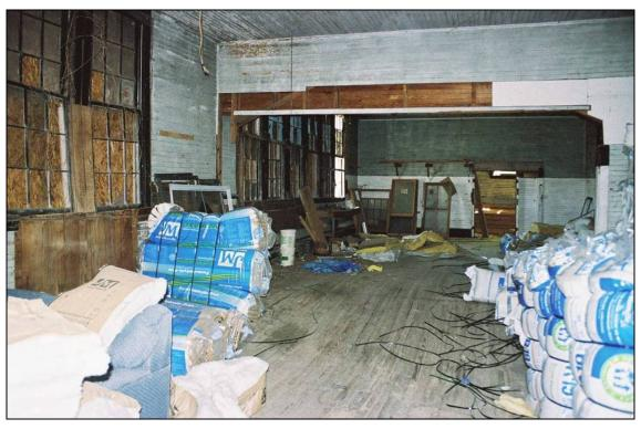
Plate 180. Jeffreys School: looking from northeast front classroom through missing partition to southeast front classroom; note banks of windows, floors, and beaded boards in place
