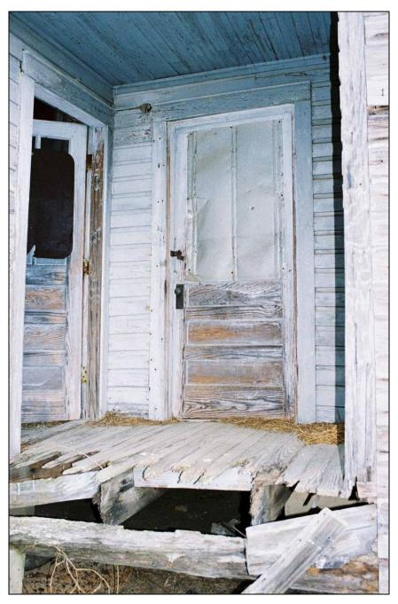
Plate 100. Springfield School: cross-panel doors to north classroom at center and industrial room on right; glass panes completely hidden by sheet metal at classroom door
