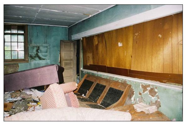
Plate 76. Chestnut School: west classroom; note original door, covered partition, and window partially obscured by dropped ceiling
