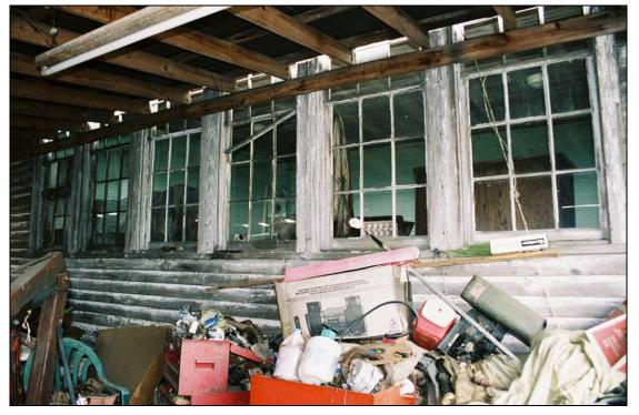
Plate 242. Dudley School: rear classroom with beaded-board walls, partition, and ceiling visible through bank of windows
