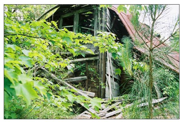
Plate 39. Lawrence School: collapsed frame; note apparently later-added paired windows in gable peak
