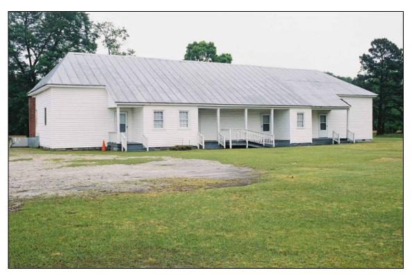
Plate 83. Marys Chapel School: south front elevation with original two classrooms at center and right and third classroom at left; note apparent removal of industrial room
