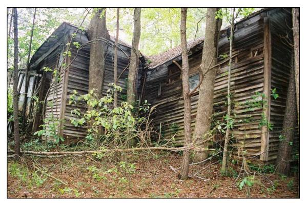
Plate 26. Coakley School: west front and south side elevations with south classroom at right and projecting cloakroom and industrial room at left
