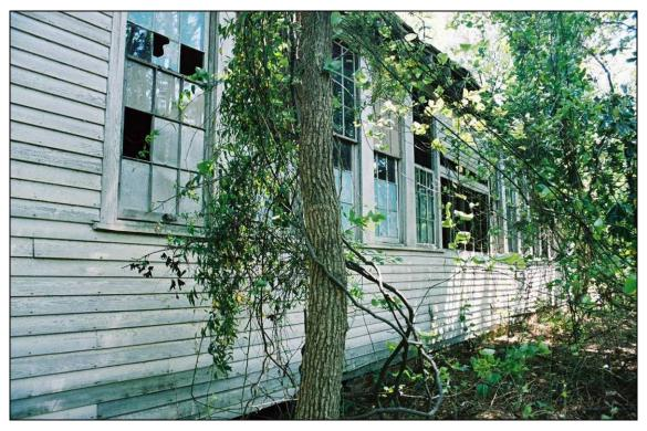
Plate 178. Jeffreys School: west rear elevation of main block; note loss of some weatherboards between the two banks of classroom windows
