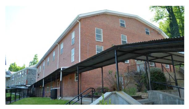
The two-story, running-bond brick, 1936 gymnasium originally featured a clipped-gable roof with exposed rafter ends and a double-leaf gable-end door sheltered by a flat-roofed bracketed canopy. Six-over-six wood sash windows, paired on the south elevation above-ground basement wall, illuminated the interior. The basement contained four classrooms. The windows and doors have been replaced and vinyl siding clads the soffits.
