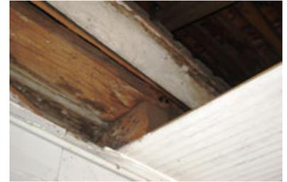
*Early cornice, exposed rafters, and wood shingles protected under the current porch roof*
