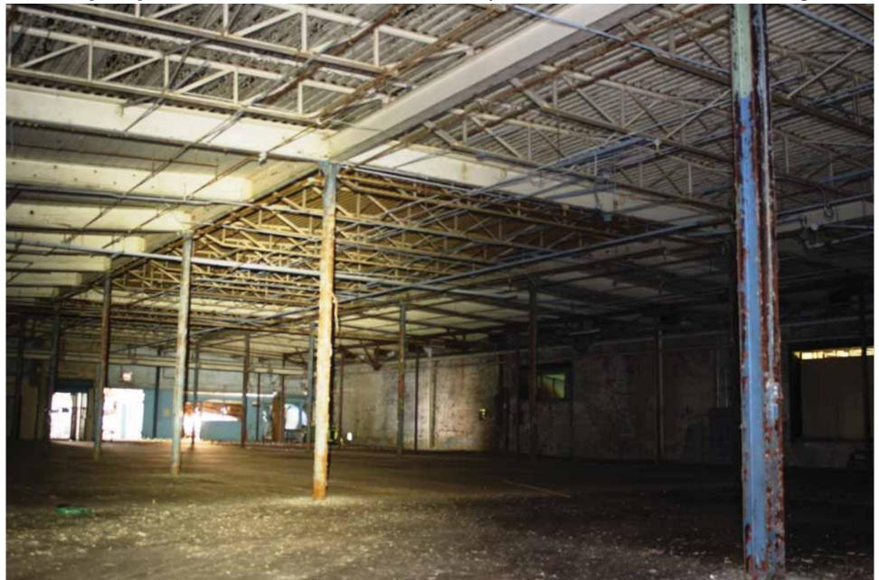
**Photo 14 of 20.** Interior of the circa 1929 addition to the Black Ox Mill (section 2), facing northeast, showing steel columns, heavy timber roof framing supplemented with steel trusses added circa 1947, and the open floor plan.
