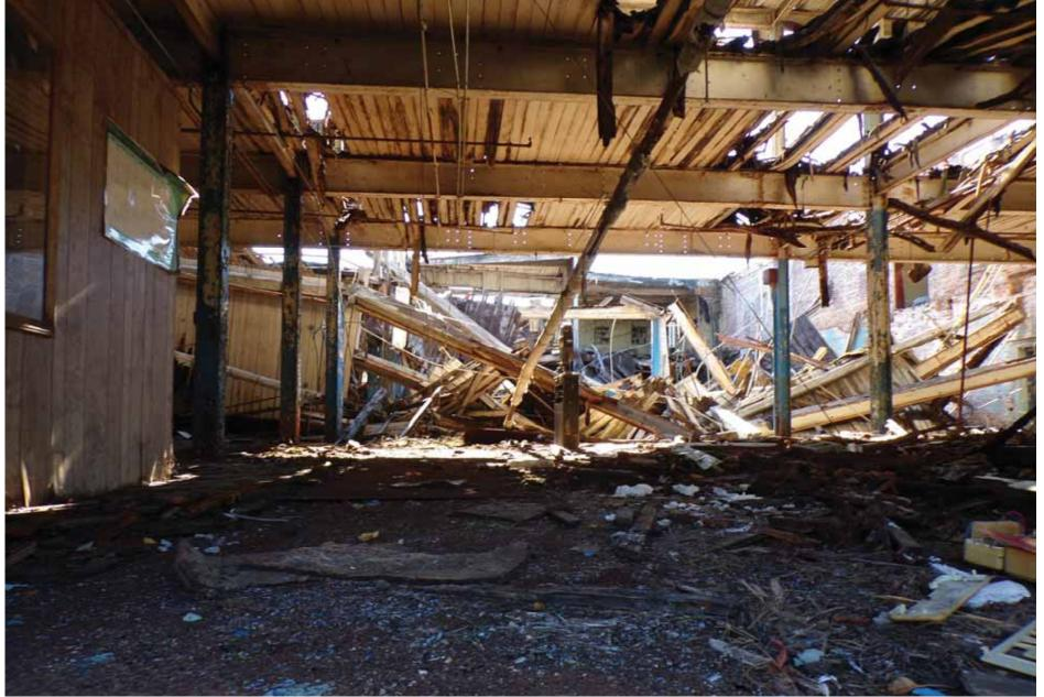
Photo 12 of 20. Interior of the 1920 Black Ox Mill (section 1), facing south, showing the collapsed roof of the two-story building.
