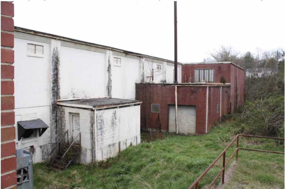
**Photo 9 of 20.** Black Ox – Duplan Corporation Mill, facing south from the west side of the property. Showing the circa 1955 addition to the west side of the 1947 addition.
