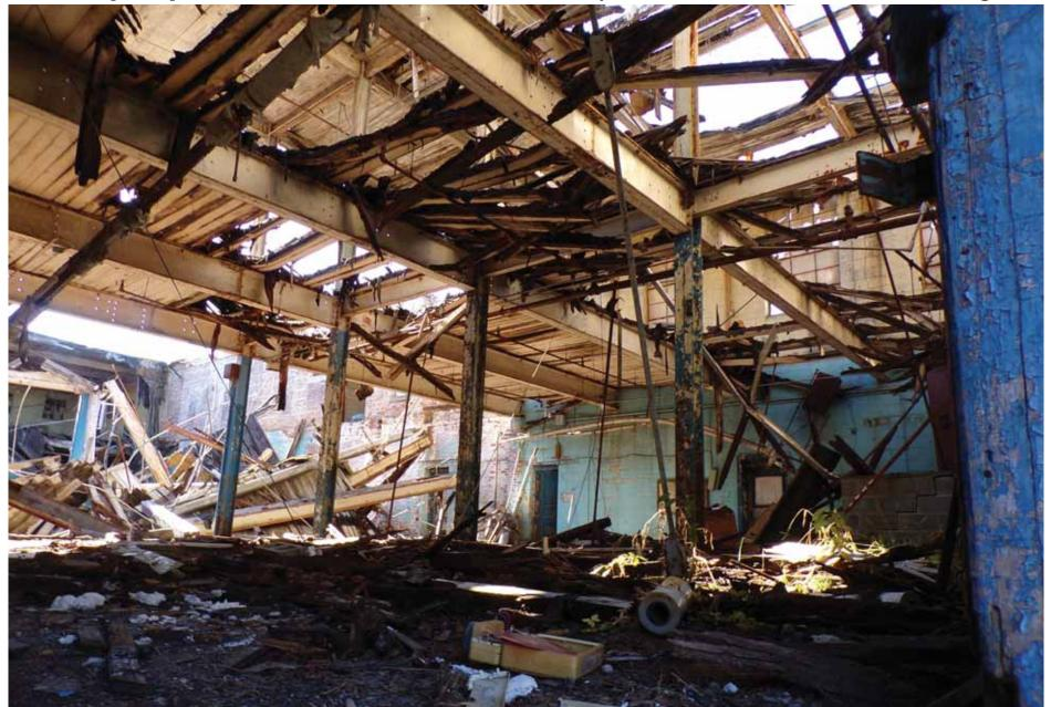
Photo 13 of 20. Interior of the two-story addition to the north side of the 1920 Black Ox Mill (section 3), facing west, showing exposed brick walls, steel framing, ceiling and floor finishes, and steel windows.
