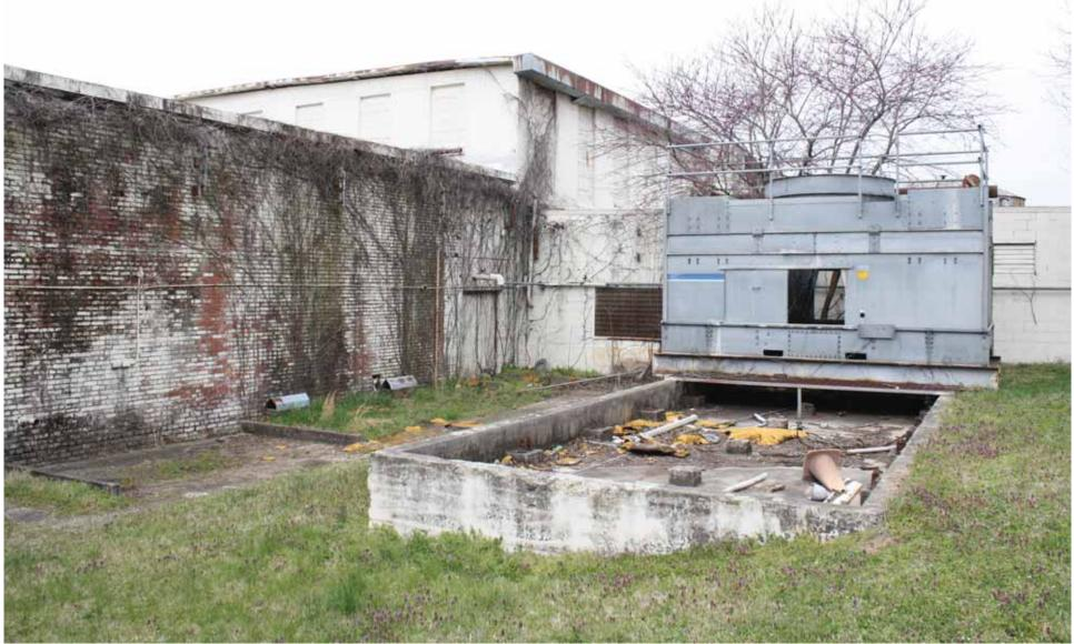
**Photo 4 of 20.** Black Ox – Duplan Corporation Mill, facing northwest from the esat side of the property. Showing the two-story 1920 mill (center), and the one-story circa 1929 addition (left). In the foreground is the foundation of a non-extant cooling tower, which now supports a circa 1980 air handling unit. Behind the unit is the one-story circa 1947 addition to the east side of the 1920 mill.
